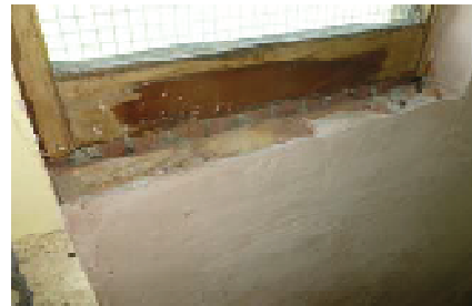
Missing internal cills and no mechanical fixings to cavity walls.
