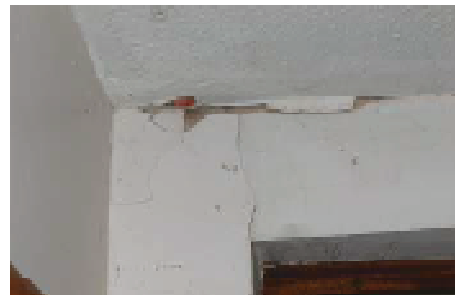
Further damage to plaster.
