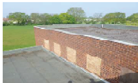
Windows removed and bricked up.
