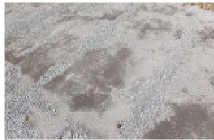
De-bonding and blistering roof coverings.
