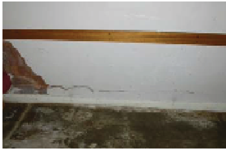
Cracking to internal walls and damaged Plaster.
