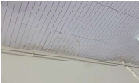
Suspended ceiling showing signs of water ingress.
