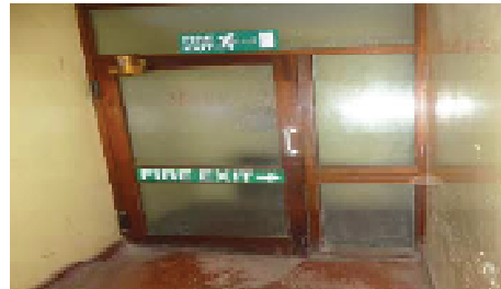
Internal doors do not have fire resisting properties.
