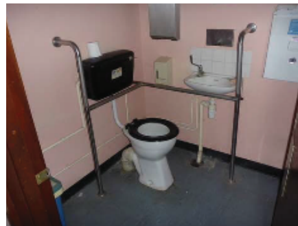
Non-compliant sanitary ware to ground floor disabled WC.
