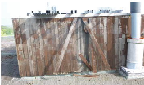
Damaged timber shiplap cladding to tank house on roof.
