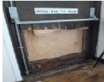
Damaged timber doors.
