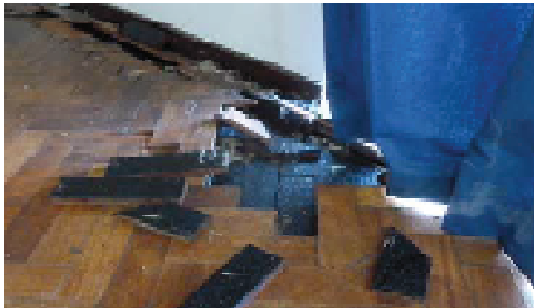
Parquet flooring uplifting to perimeter of the main hall.
