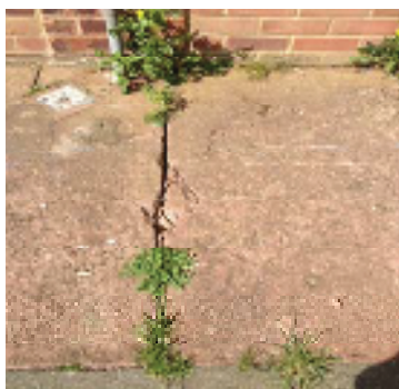
Cracking to footpath and uneven surfaces.
