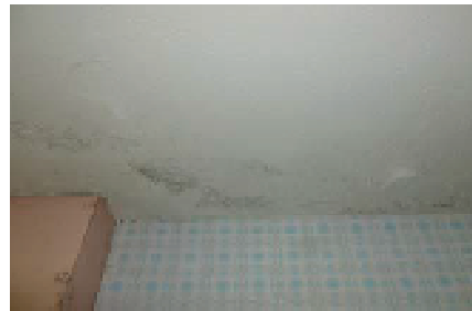
Friable textured coated ceilings. Also signs of water ingress and mould growth.
