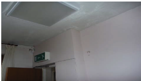
Asbestos containing artex has become friable. Encapsulate & decorate as a minimum.
