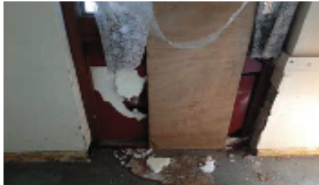
Damaged doors and missing/ broken glazing.
