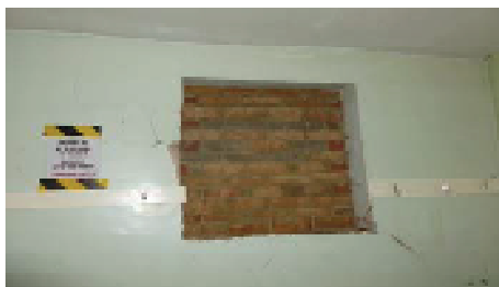
Internal view of blocked up windows blocking light and natural ventilation.
