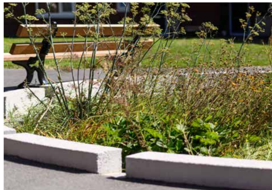
Fig 6.48 - Example of street rain garden, Victoria Crescent, Seven Sisters. Credit: Robert Bray Associates
