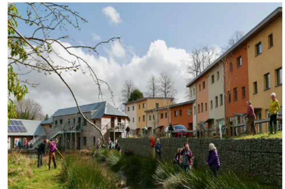
Fig 6.49 - Example of multi-functional attenuation basin, Cannock Mill Co-Housing, Colchester. Credit: Robert Bray Associates
