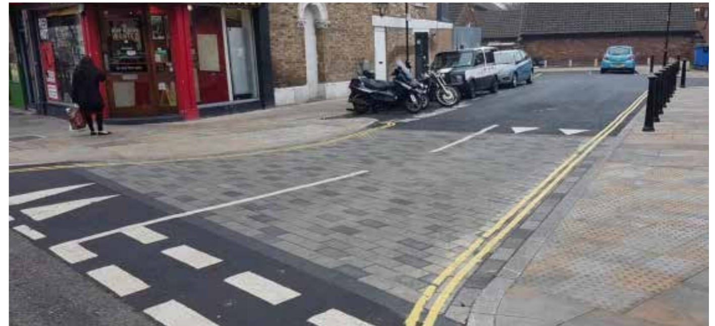
Fig 6.19 - Copenhagen Crossing. Credit: Create Streets
