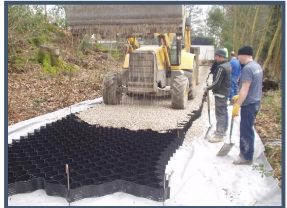
Figure 10 Examples of Cellweb filling with angular stone
