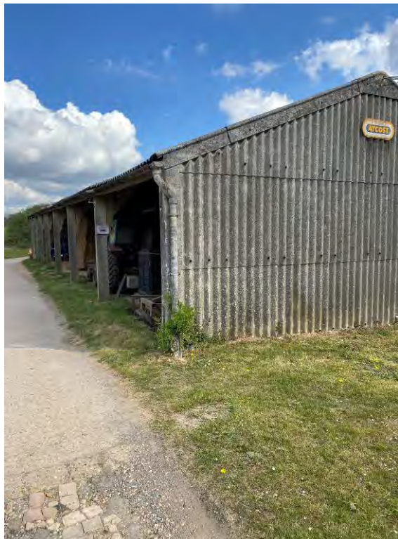
Photo 3 – Suspected cement bound asbestos cladding on barn behind residential bungalow on Cook's Land.
