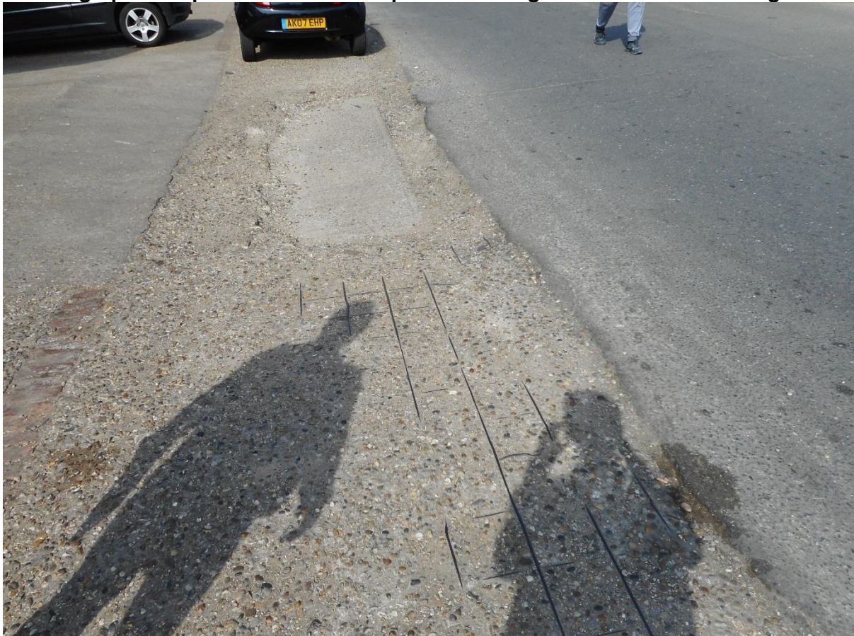
Photograph 2: Exposed metalwork at point of damaged surface in Armstrong Road
