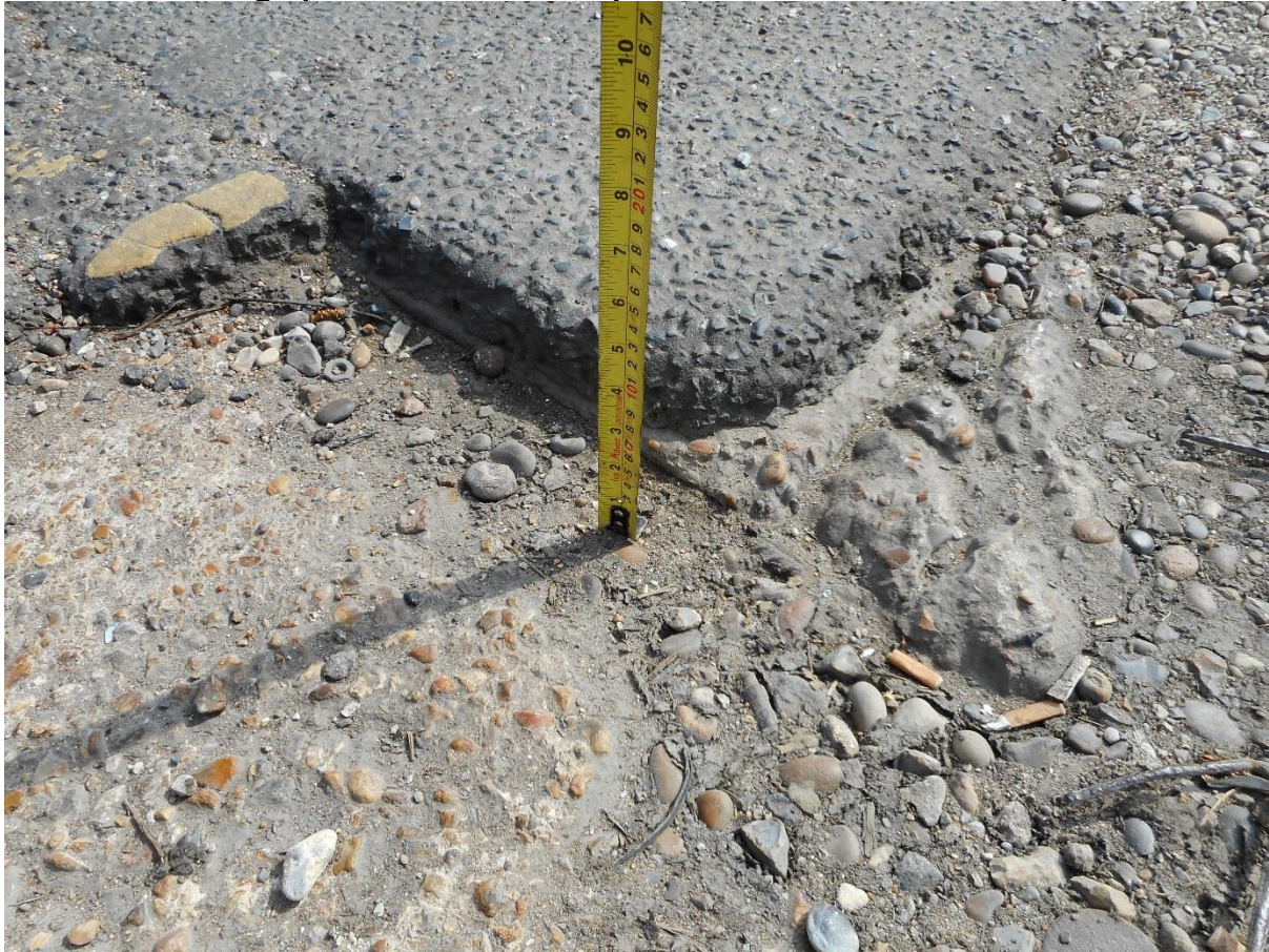
Photograph 5: Pot hole with tape measure to demonstrate depth
