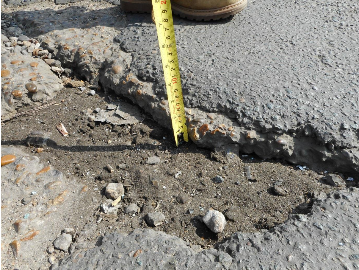
Photograph 15: Example of pot hole demonstrating depth and road surface quality
