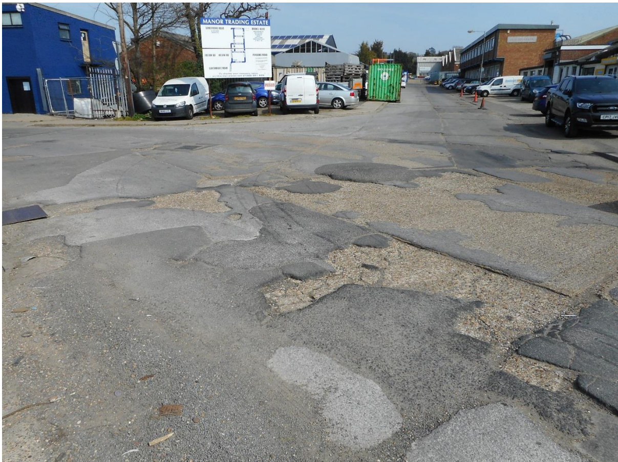
Photograph 4: Junction of Armstrong Road and Brunel Road showing dilapidated condition of road surface
