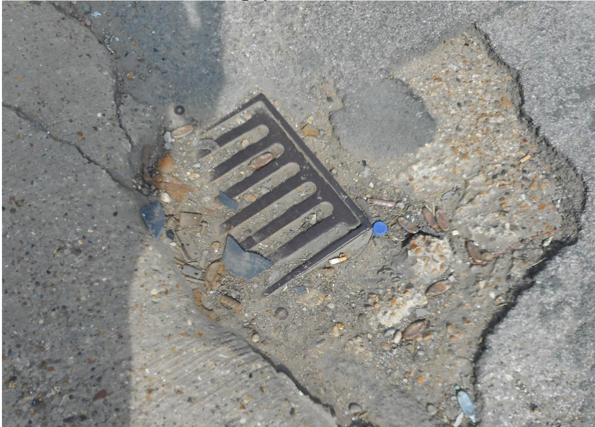
Photograph 3: Blocked drain
