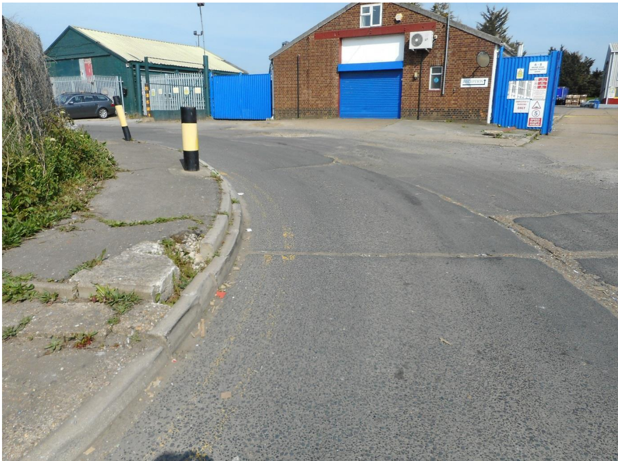
Photograph 14: Poor condition of corner of Brunel Road with damaged footway, kerb, bollard and road surface evident
