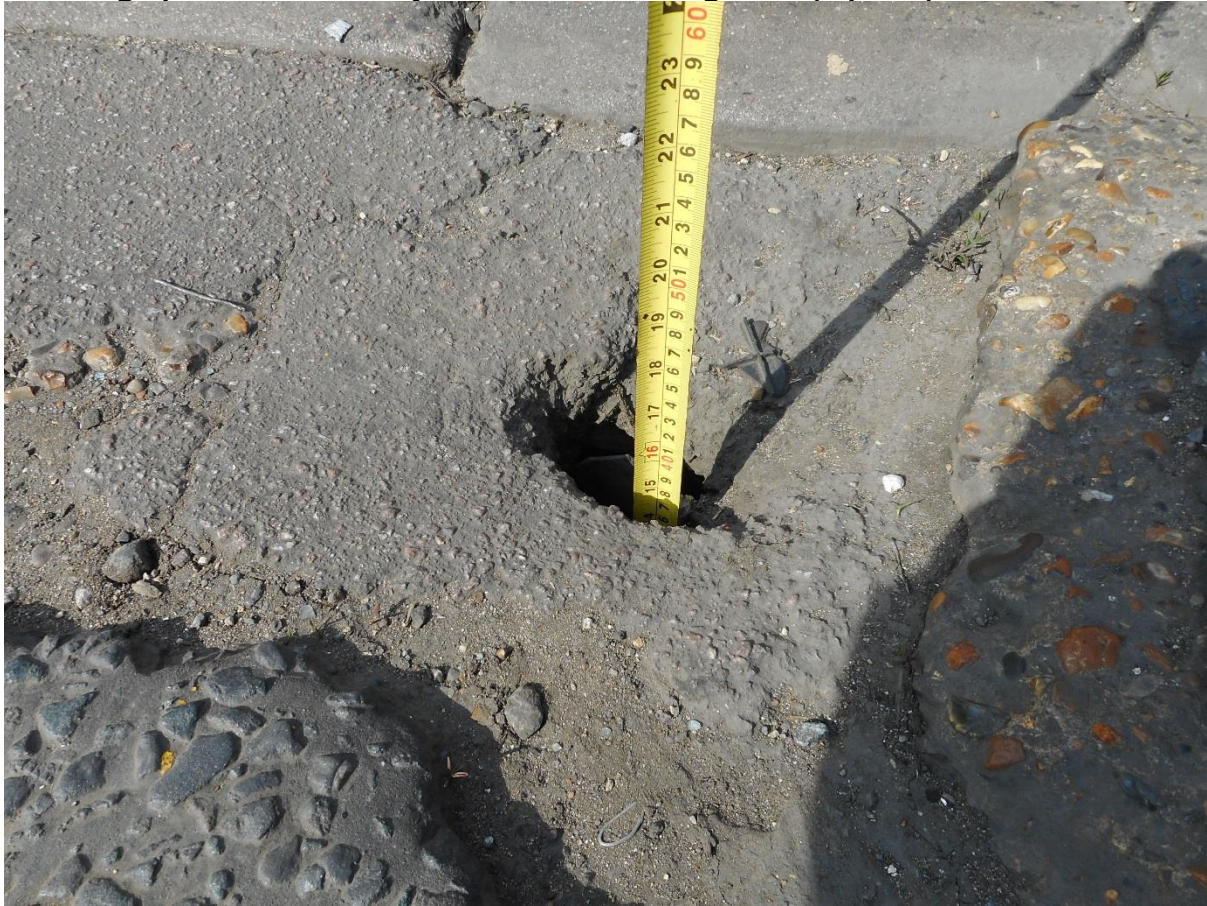
Photograph 9: Sink hole at junction of Armstrong Road (top end) and Brunel Road
