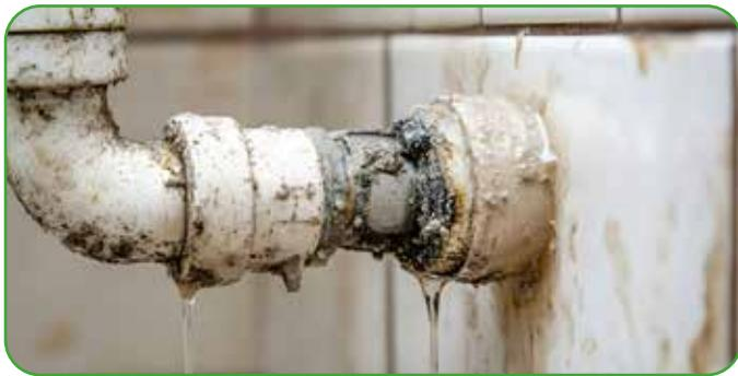
Leaks from water and waste pipes in the home are common, especially in bathrooms and kitchens. With traumatic damp you will see an area or patch of damp that looks and feels wet. Black mould does not normally develop with traumatic damp because chemicals in the water prevent it growing.
