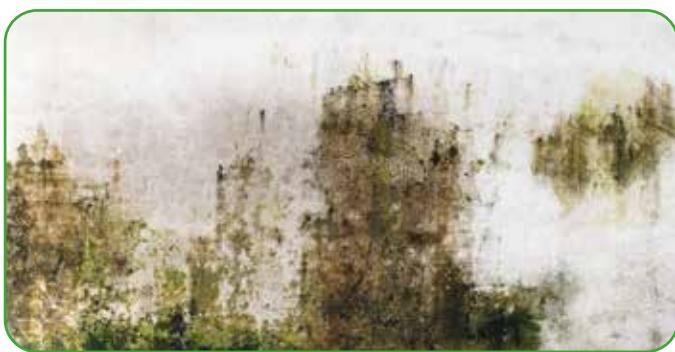
Occurs when water in the ground enters a property by travelling up through the pores in brickwork, usually due to a broken or missing damp proof course. Rising damp only affects basements/cellar rooms and ground floor rooms. It usually leaves a brown 'tide' mark caused by salts from the ground. Black mould does not normally develop with rising damp because the salts prevent it growing.
