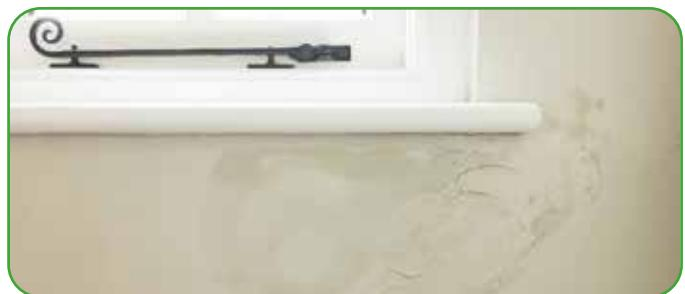
Penetrating damp is caused by water passing through the external walls or roof of a house because of a problem such as missing roof tiles, damaged pointing to brickwork, or cracked render. It is only found on external walls and sometimes on ceilings if there is damage to the roof.
